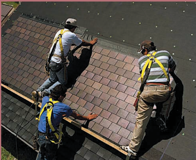
Figure 3: Photovoltaic modules in the form of shingles for roof integration. (Photo: Warren Gretz)
