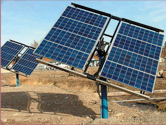
Figure 2: A mechanical tracking system keeps solar cells facing the sun, thereby capturing more of the available solar energy. (Photo: National Center for Appropriate Technology)
